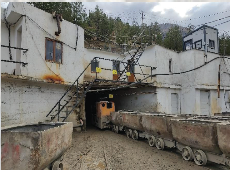
Fig.7 Main Level 41 Entrance Bulqiza North
