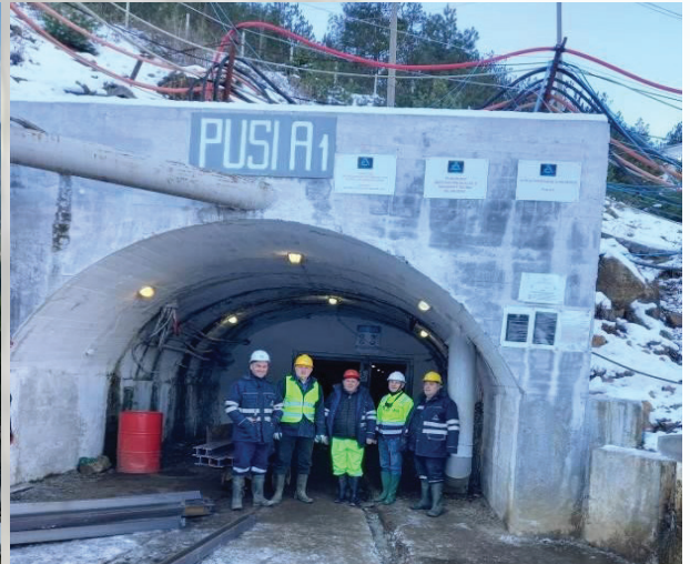
Fig. 6 Shaft A1 Entrance Bulqiza North
