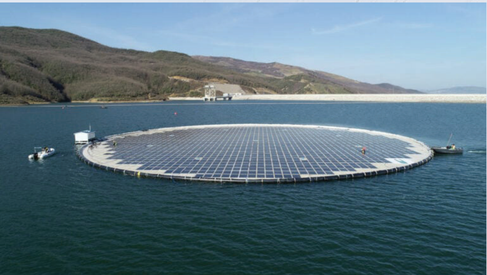
Fig. 7. Floating Photovoltaic Plant on Banja Lake
